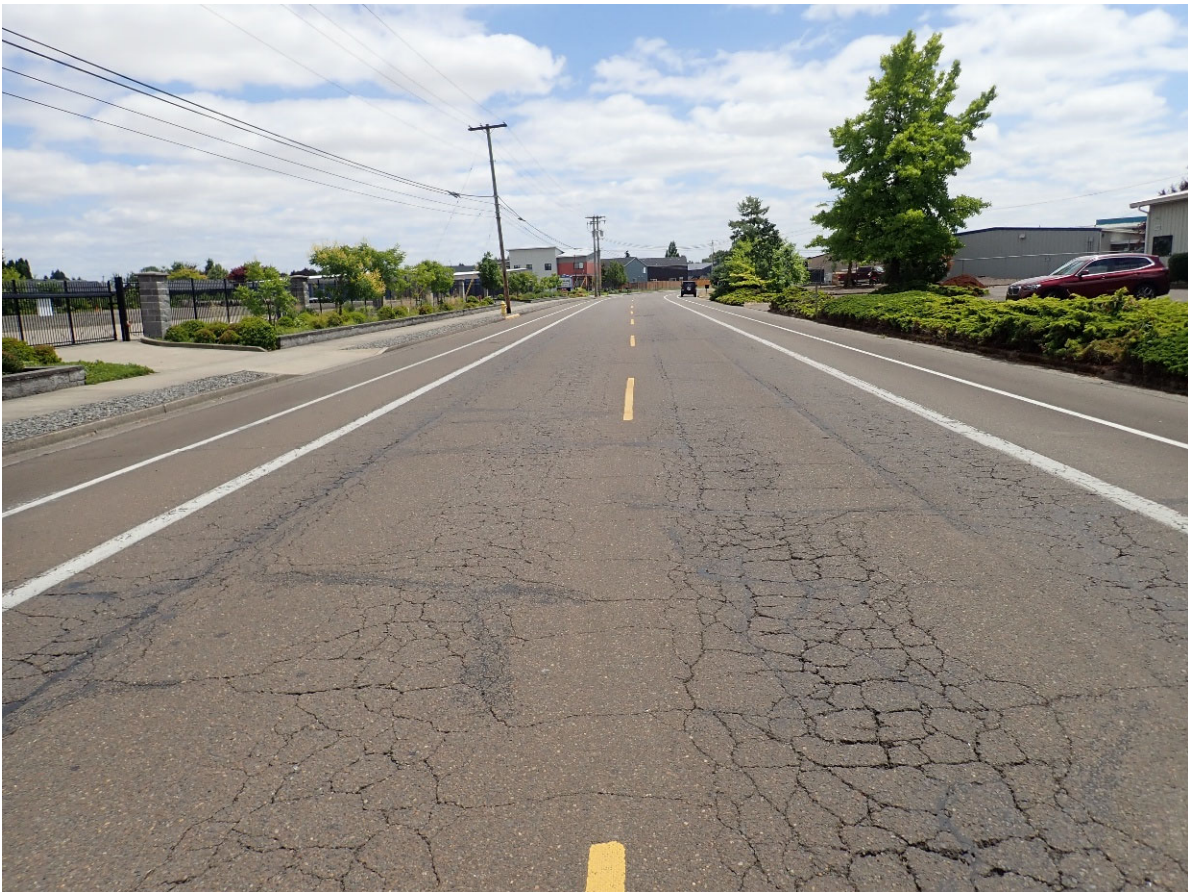
8. Looking southbound from 125 feet south of 25 th Avenue SW.
