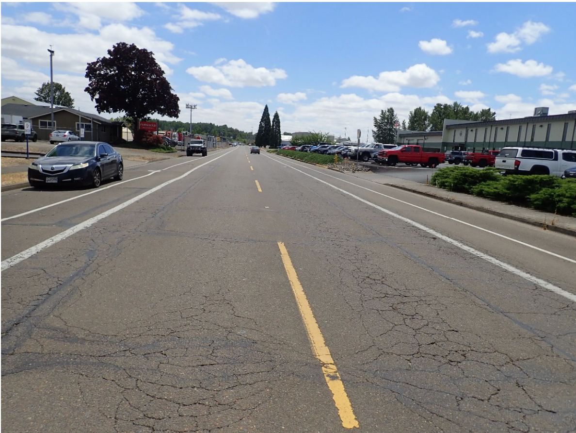
10. Looking southbound from 450 feet south of 29 th Avenue SW.
