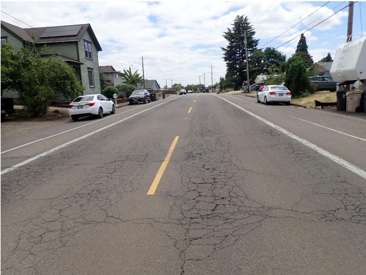
4. Looking southbound from 200 feet south of 20 th Avenue SW.
