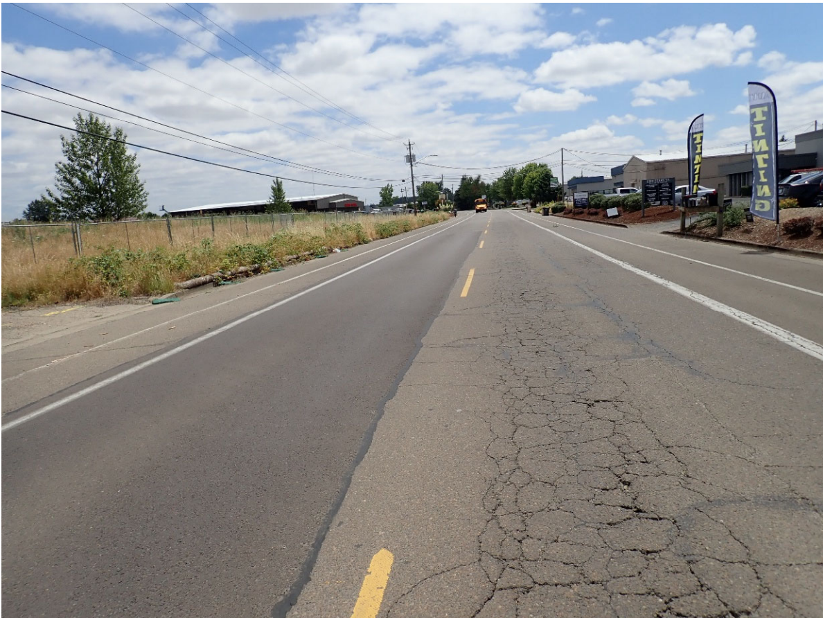
6. Looking southbound from 350 feet south of 22 nd Avenue SW.
