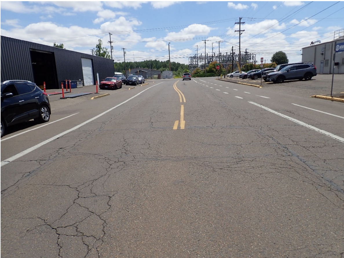
12. Looking southbound from 250 feet north of 34 th Avenue SW.
