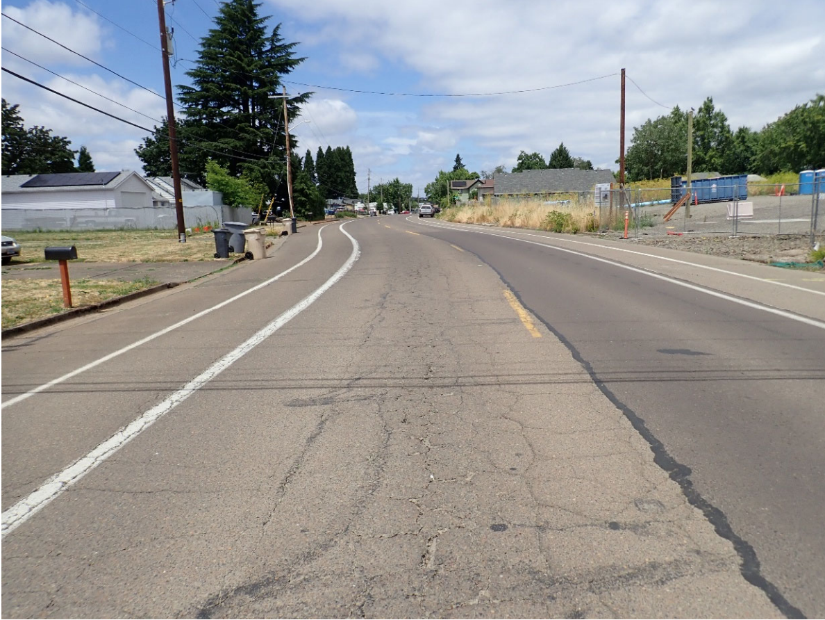
5. Looking northbound from 350 feet south of 22 nd Avenue SW.
