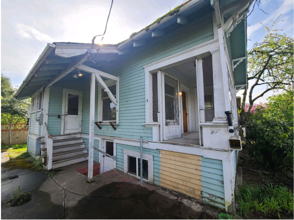
North side of subject house before temporary steps were installed
