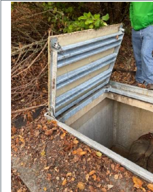
Photo 4-2-3 Broadway – Valve Vault - FRP Hatch
