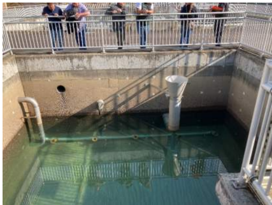
Photo 4-3-9 A&M WTP – Coat Exposed Aggregate in Neutralization Basin
