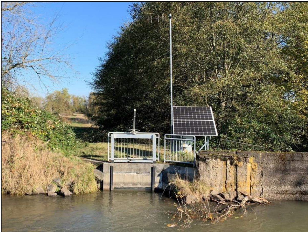
Figure 5. Cox Creek Diversion
