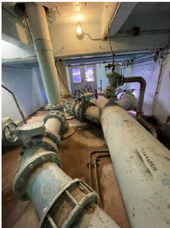
Photo 4-4-20 Vine St – FWPS Pipe Gallery – Corrosion & Rust
