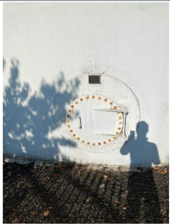
Photo 4-3-36 Maple Street Reservoir
