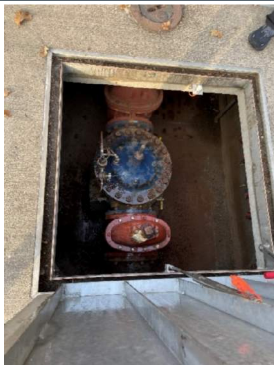
Photo 4-4-2 Broadway – Valve Vault – Rusty Piping
