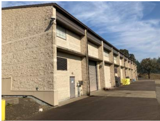
Photo 4-3-7 A&M WTP – Clear Gutters, Clean & Seal CMU Wall
