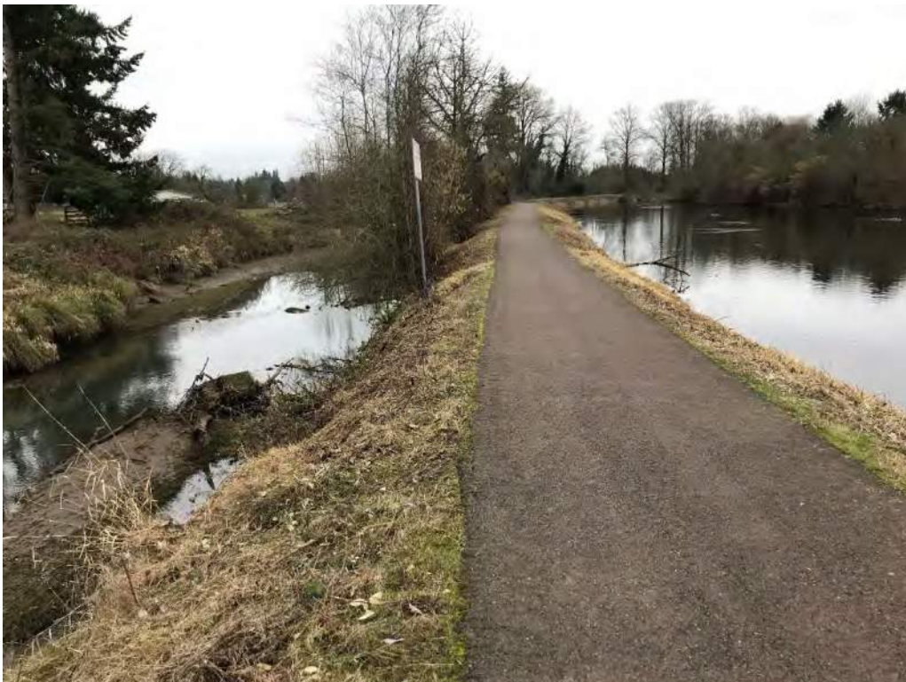
Photo 2. View of berm at Point B (Figure 1) facing southeast.
