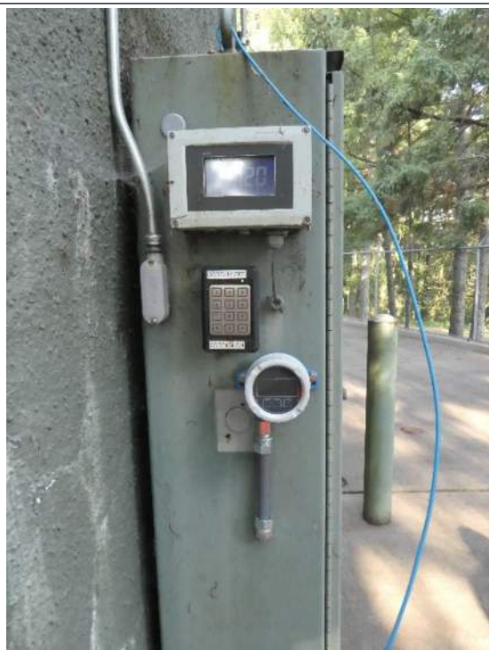
Photo 4-5-10 Wildwood – Level Sensor Transmitter
