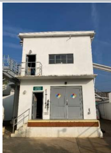
Photo 4-3-12 Vine WTP – Control/ Chemical Storage Building
