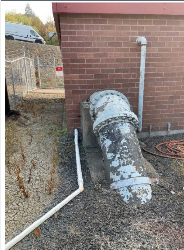
Photo 4-4-8 North Albany – Exterior PS Piping – Chipped Coating
