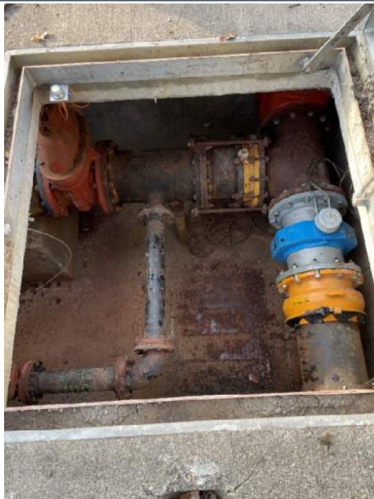
Photo 4-4-1 34 th St PS- Piping - Add Pipe Supports
