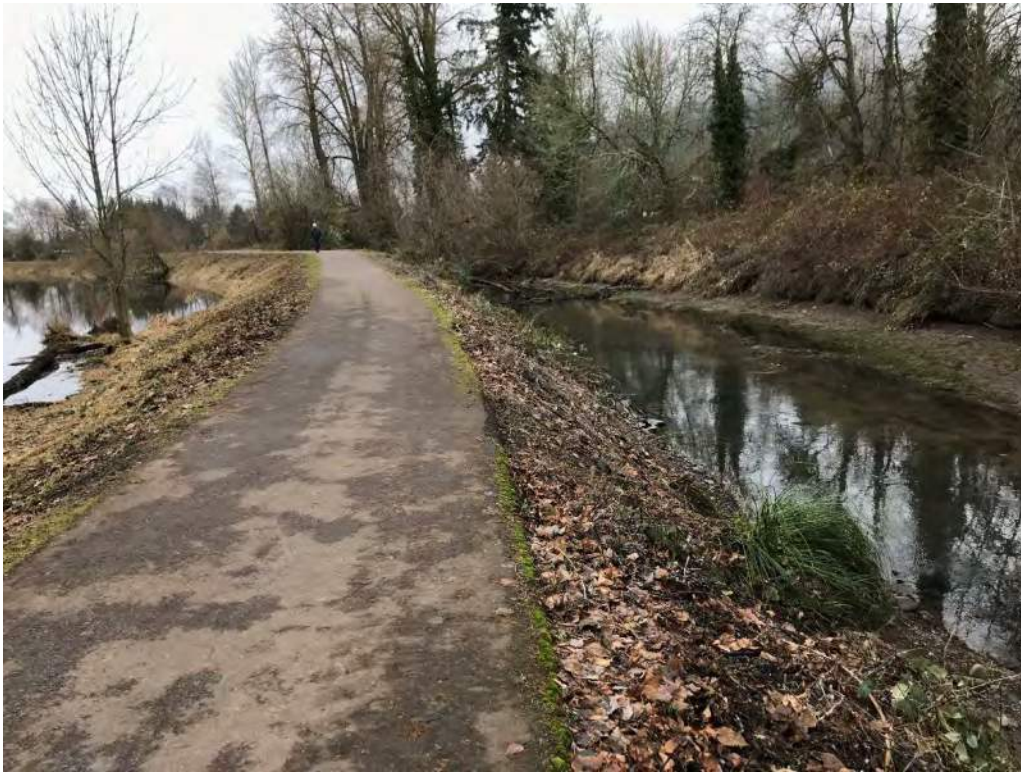
Photo 1. View of the berm at Point A (Figure 1) facing northwest.
