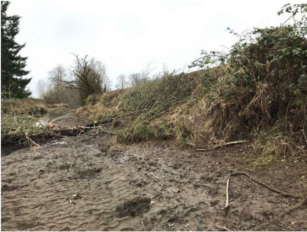
Photo 5. Typical steep berm slope along the canal facing southeast.
