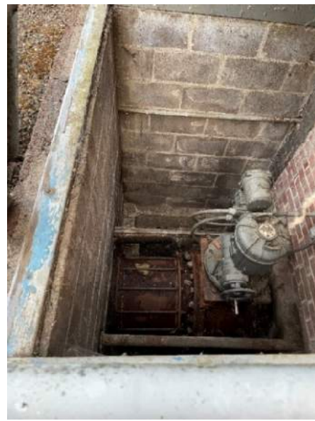
Photo 4-2-10 Vine St – RWPS Valve Vault – Made of CMU
