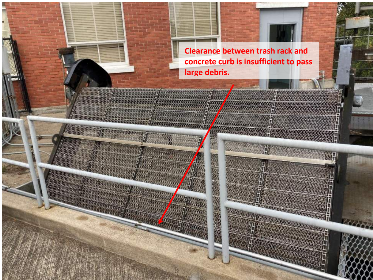
Figure 2. A View of the Upstream Side of the Trash Rack Showing Little Clearance for Large Debris Removal
