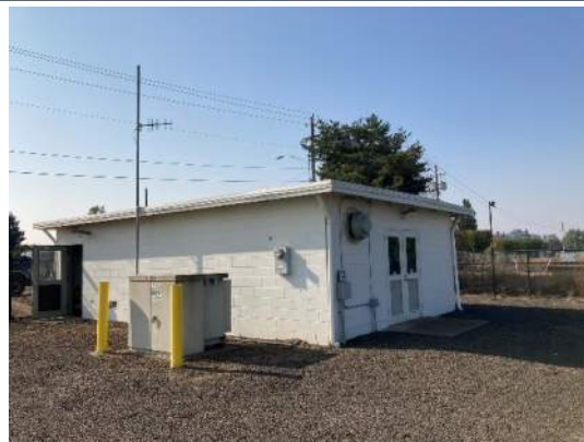
Photo 4-3-23 34th Street Pump Station
