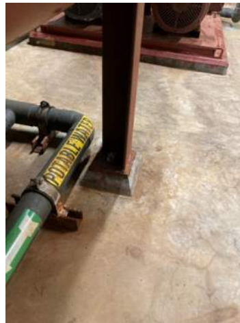
Photo 4-3-8 A&M WTP – Remove Rust & Recoat Metal
