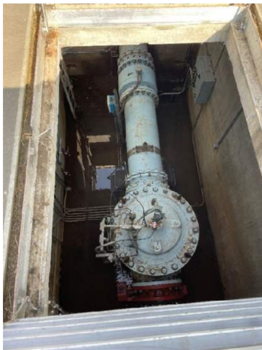
Photo 4-2-9 Vine St – RWPS Meter Vault – Standing Water
