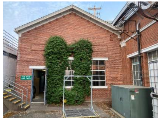
Photo 4-3-10 Vine WTP – Raw Water Intake Pump Station
