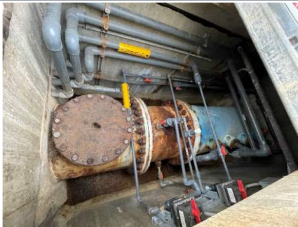
Photo 4-4-20 Vine St – FWPS Pipe Gallery – Corrosion & Rust
