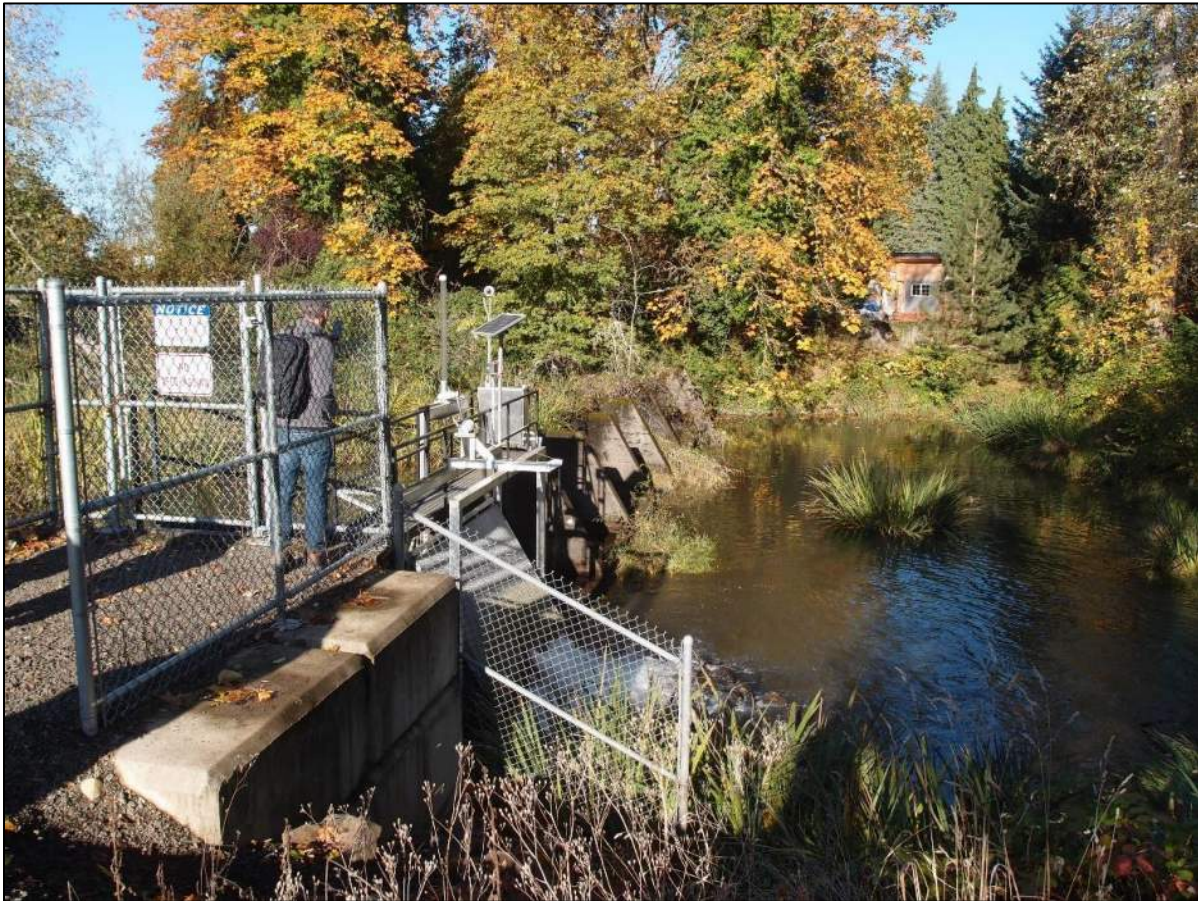
Figure 3. Mark's Slough Diversion
