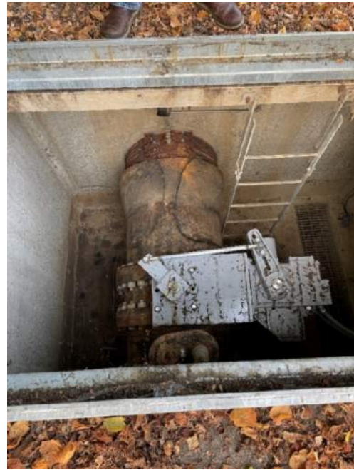
Photo 4-4-2 Broadway – Valve Vault – Rusty Piping
