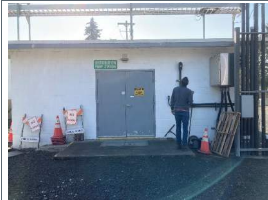
Photo 4-3-19 Maple Pump Station
