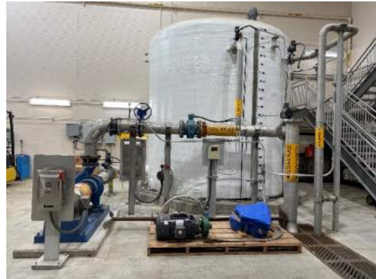
Photo 4-6-6 Vine St - Chemical Room – Add tank anchorage and MSDS
