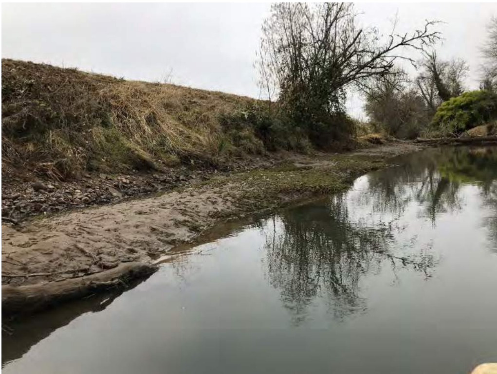
Photo 4. Typical steep berm slope along canal facing west.
