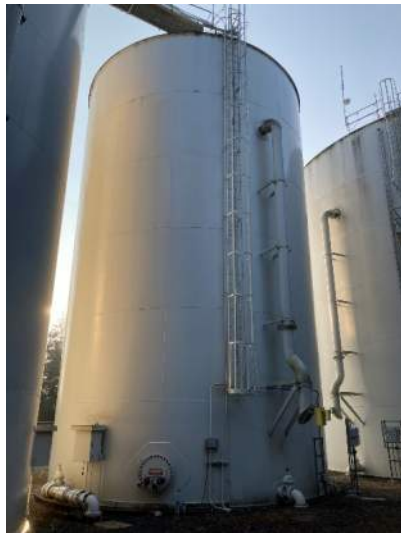
Photo 4-3-27 Valley View Reservoir
