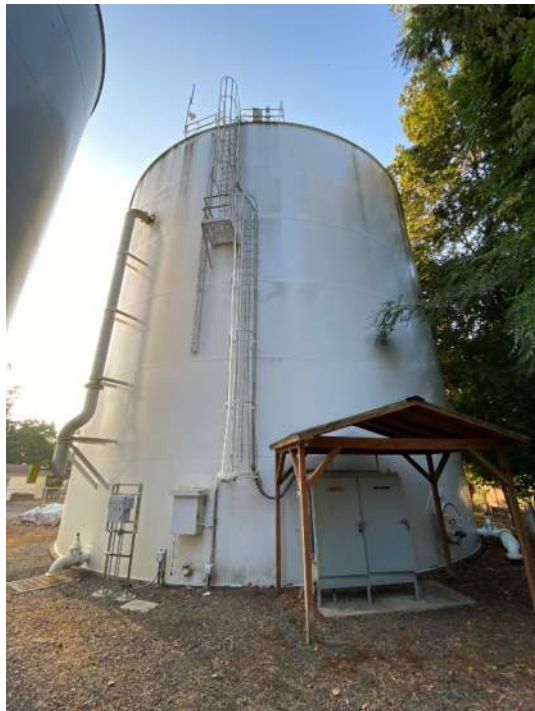
Photo 4-3-33 Valley View Reservoir
