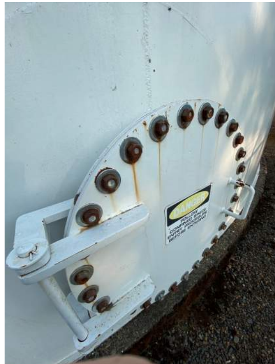
Photo 4-3-34 Valley View Reservoir
