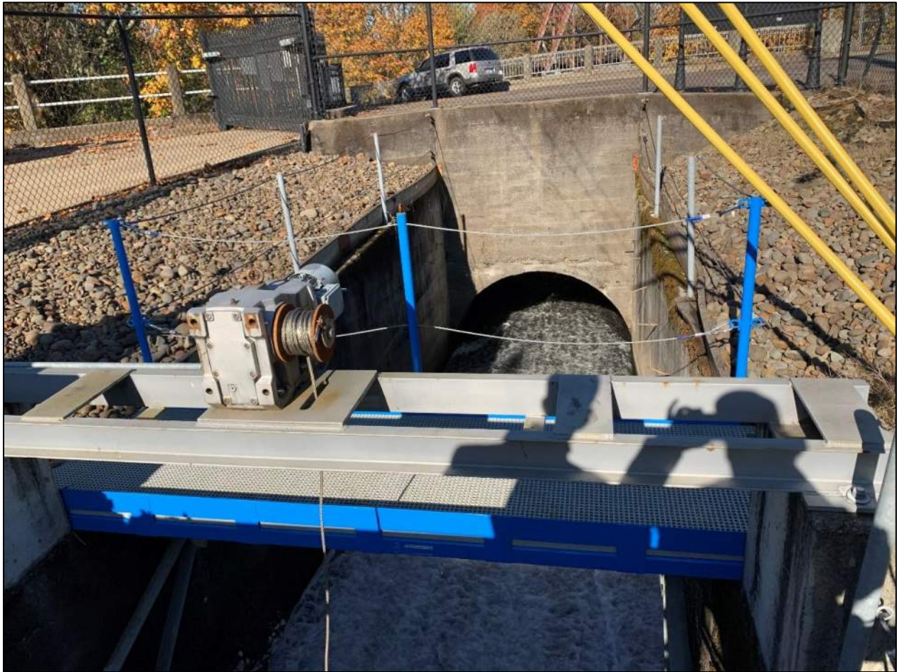
Figure 6. Vine Street Radial Gate Operator and Outfall
