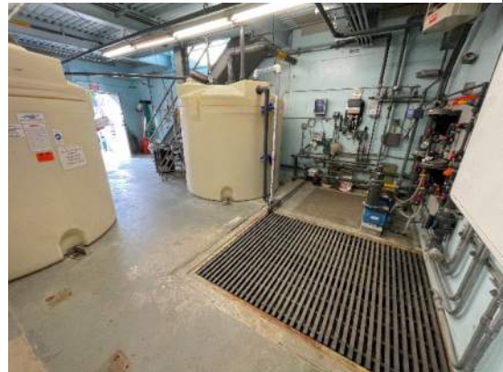
Photo 4-6-6 Vine St - Chemical Room – Add tank anchorage and MSDS
