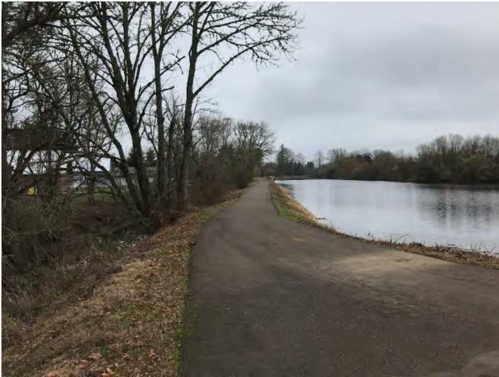
Photo 3. View of berm at Point C (Figure 1) facing southeast.
