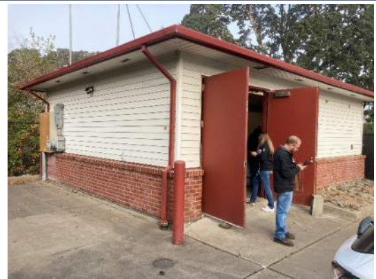
Photo 4-3-24 Gibson Hill Pump Station
