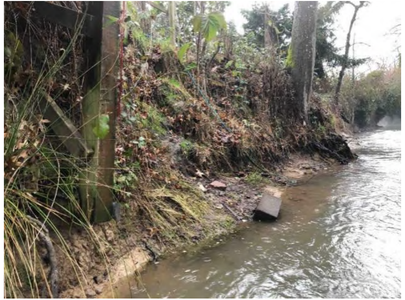
Photo 1010: Upstream toward right bank
