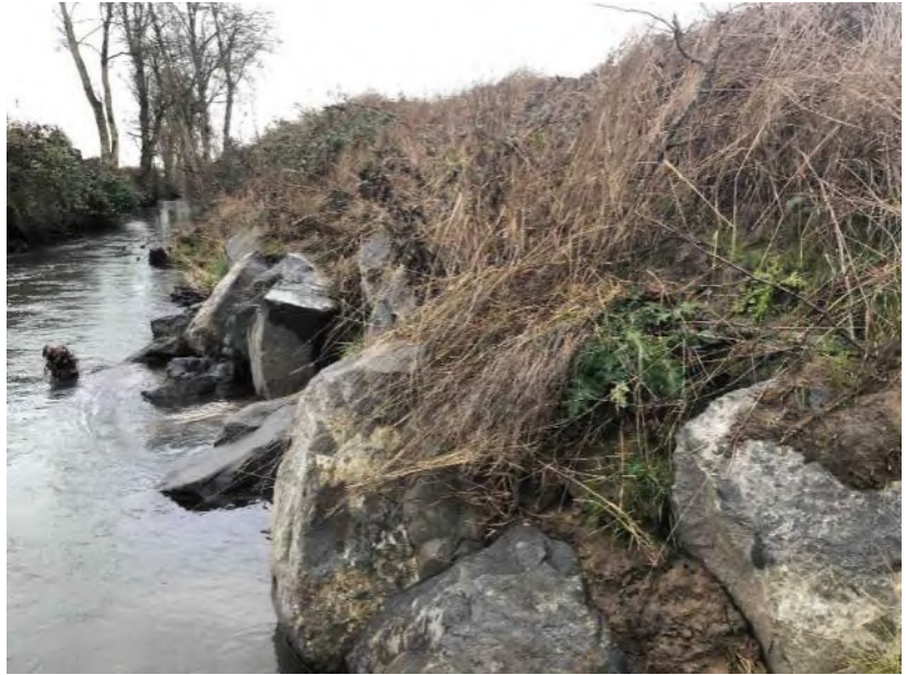
Photo 787: Right bank with Riprap
