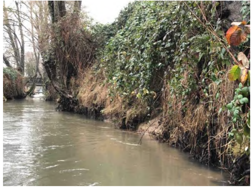
Photo 879: Downstream towards right bank
