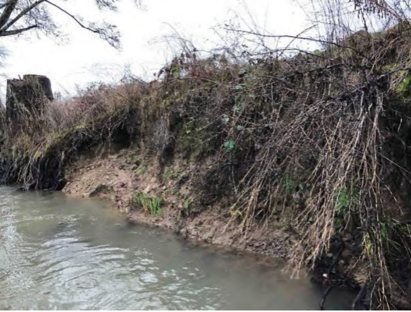
Photo 914: Upstream toward left bank
