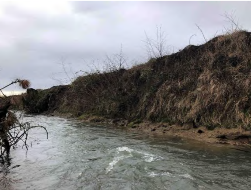
Photo 769: Upstream to Downstream panorama of right bank
