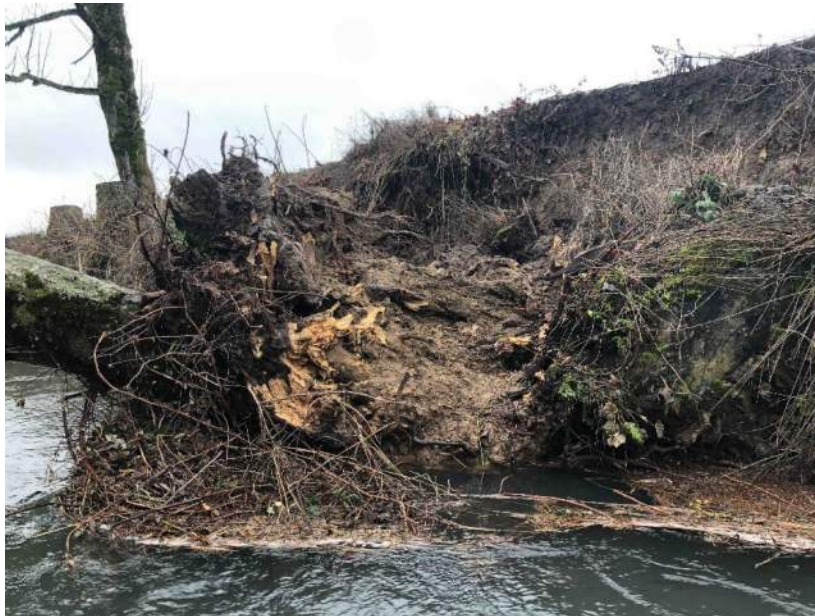
Photo 795: Upstream toward left bank
