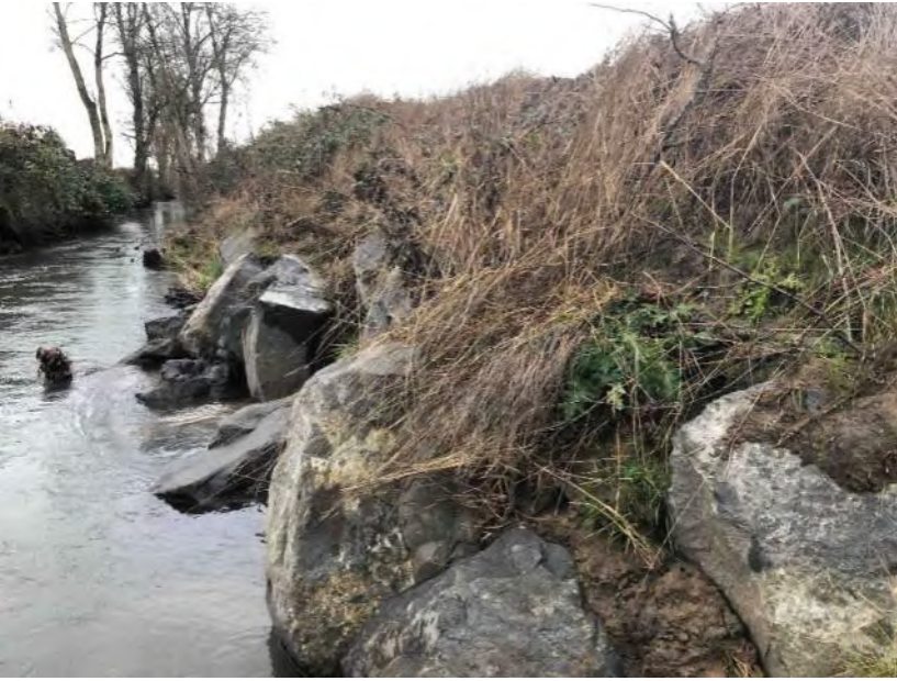
Photo 787: Downstream towards right bank
