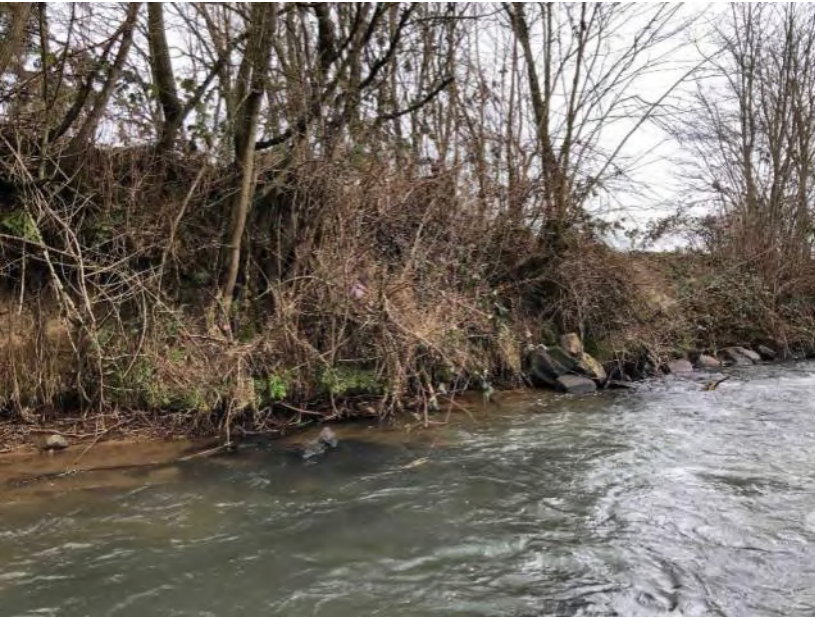
Photo 624: Downstream to upstream panoramic view of right bank
