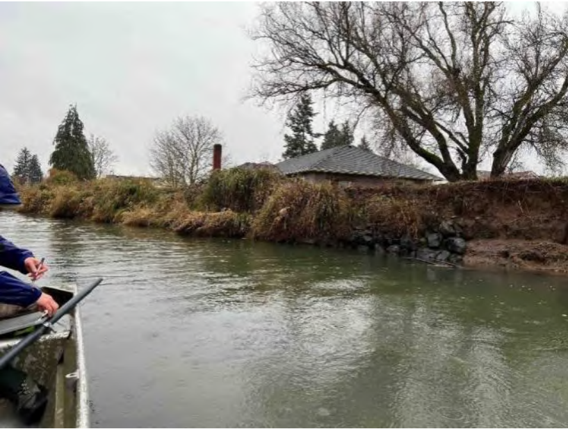
Photo 2916: Upstream to downstream panorama of right bank
