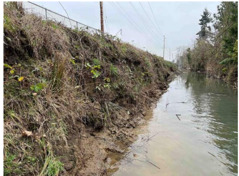
Photo 3079: Upstream toward right bank
