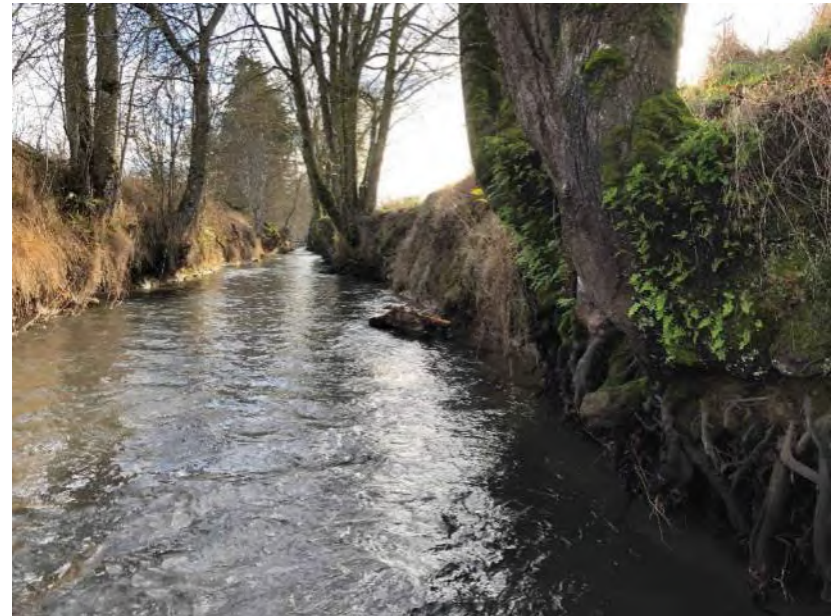
Photo 561: Upstream toward left bank
