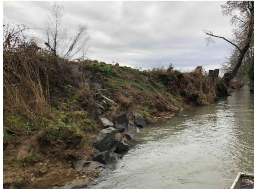
Photo 893: Downstream toward left bank, note riprap protecting small outfall
