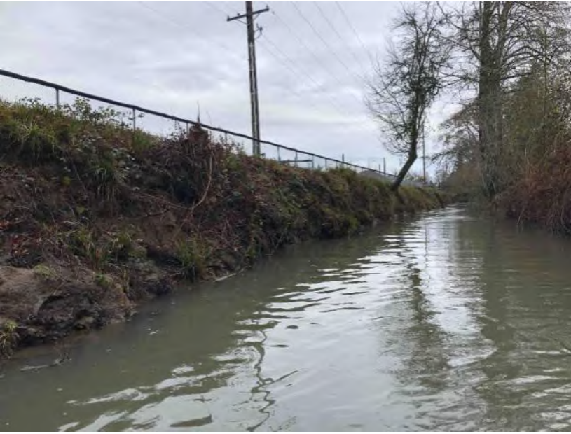
Photo 975: Upstream toward right bank
