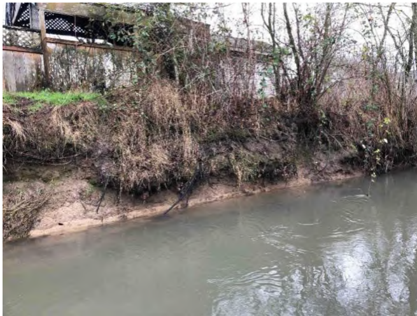
Photo 946: Upstream to downstream panorama of right bank
