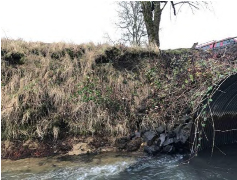
Photo 767: Upstream to Downstream panorama of right bank
