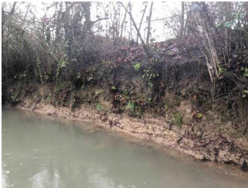
Photo 997: Upstream toward left bank
