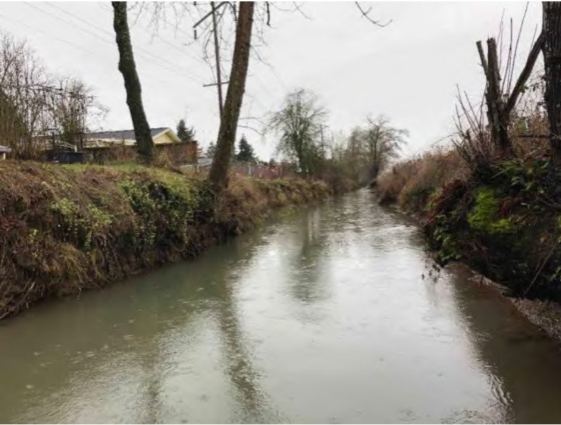
Photo 923: Upstream, see also right bank erosion upstream of tree
