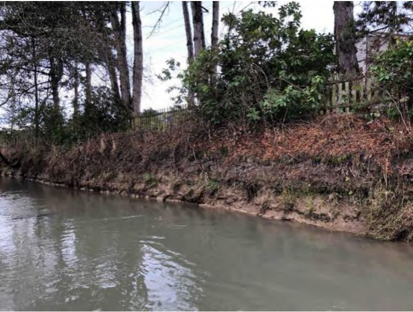
Photo 948: Upstream to downstream panorama of right bank
