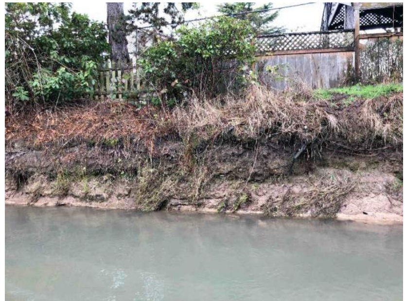
Photo 947: Upstream to downstream panorama of right bank
