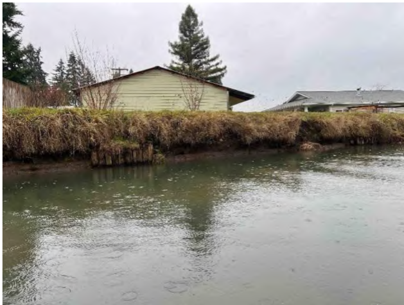
Photo 2915: Upstream to downstream panorama of right bank
