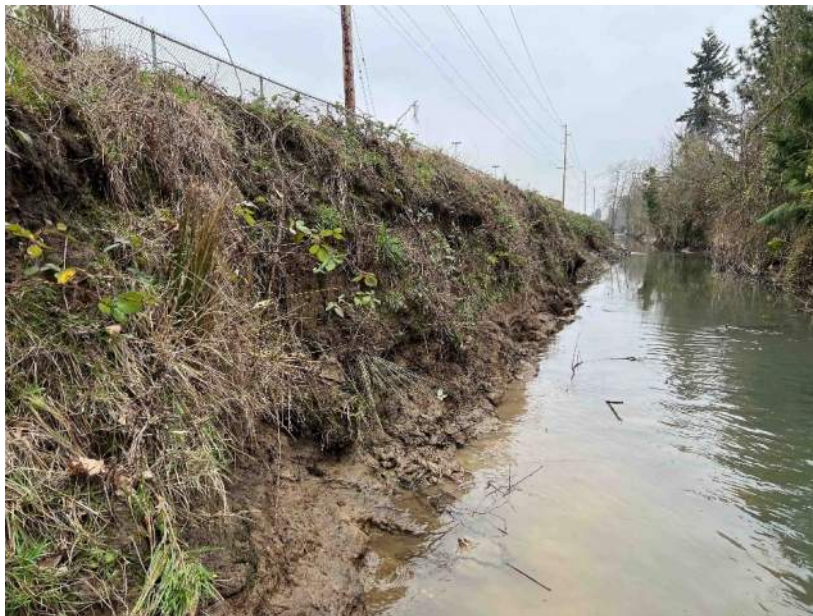
Photo 3079: Upstream toward right bank
