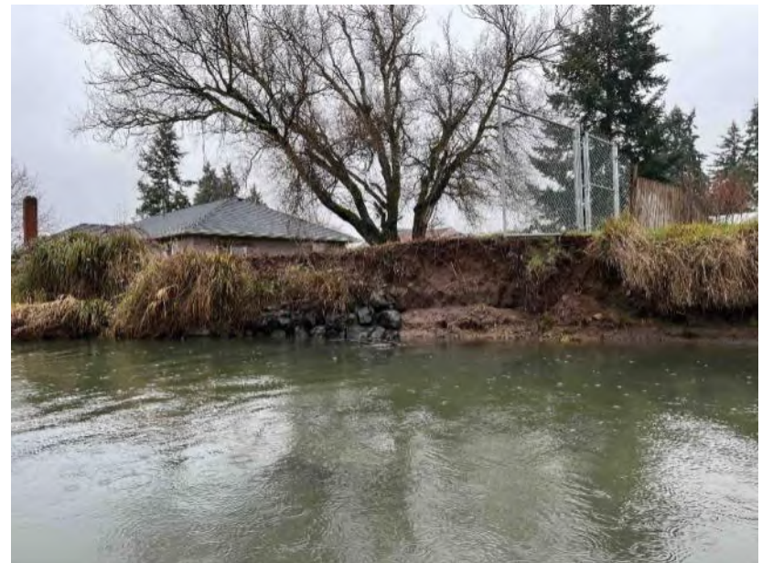
Photo 2914: Upstream to downstream panorama of right bank
