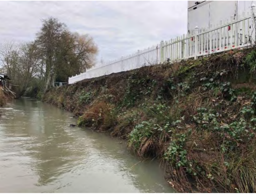
Photo 857: Upstream toward left bank
