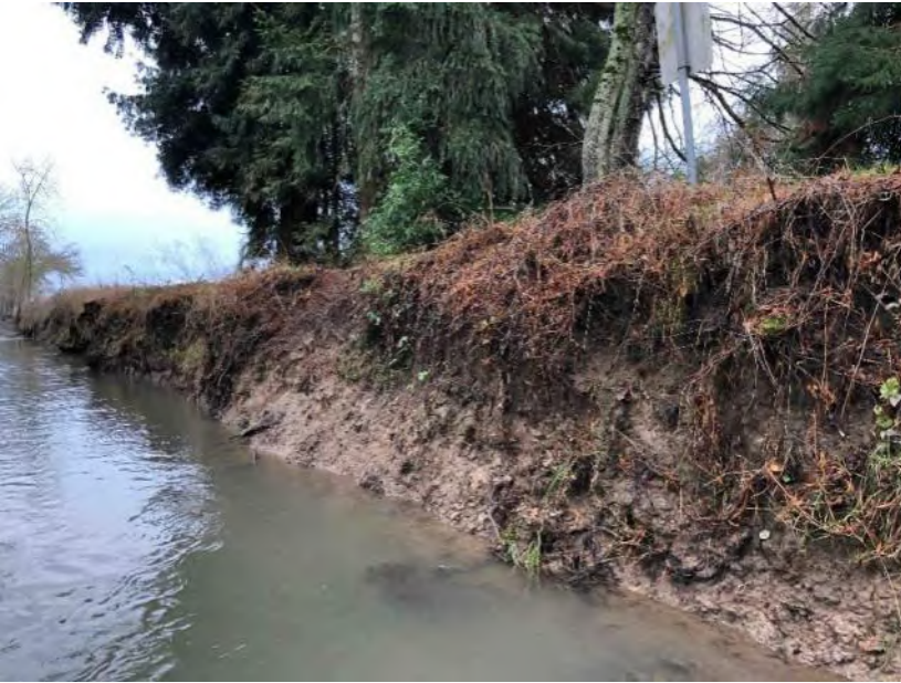
Photo 939: Upstream toward left bank
