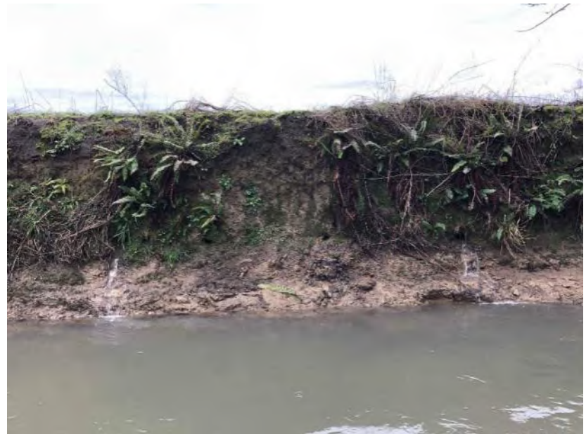
Photo 898: Upstream to downstream panorama
