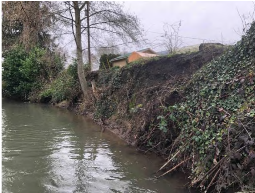
Photo 823: Downstream towards right bank
