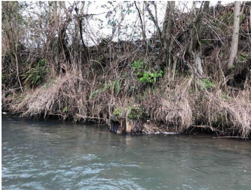
Photo 622: Downstream to upstream panoramarama of right bank
