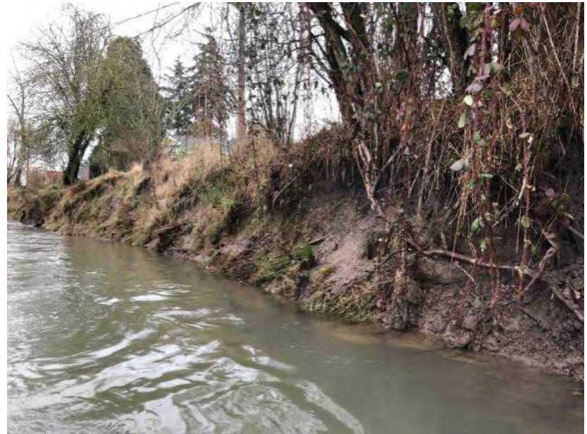
Photo 921: Downstream towards right bank
