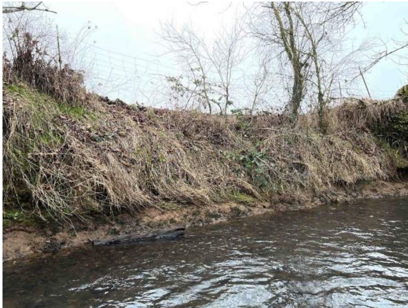
Photo 3057: Left bank failure
