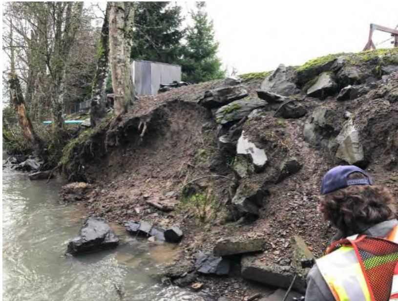
Photo 847: Upstream toward left bank
