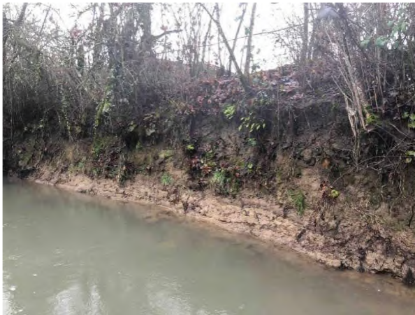
Photo 997: Upstream toward left bank
