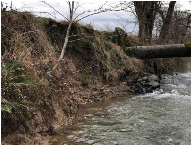
Photo 687: Upstream toward right bank
