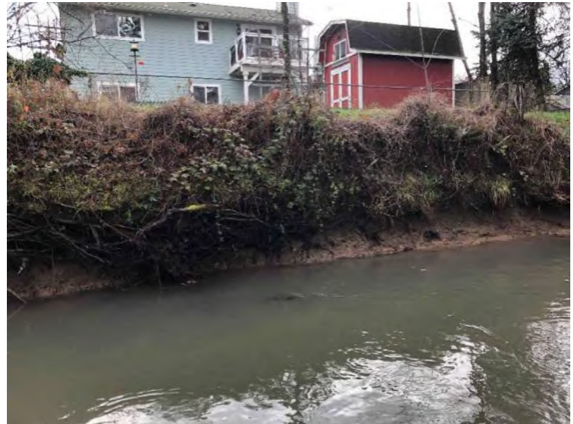
Photo 943: Downstream towards left bank (undercut downstream of site)
