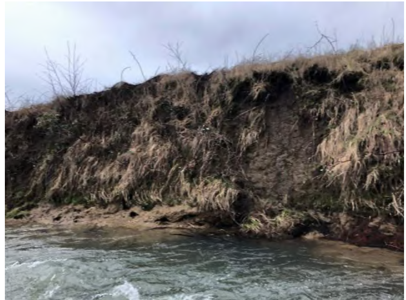
Photo 768: Upstream to Downstream panorama of right bank
