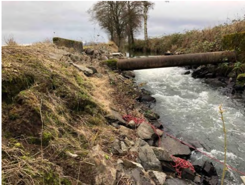
Photo 667: Upstream toward right bank
