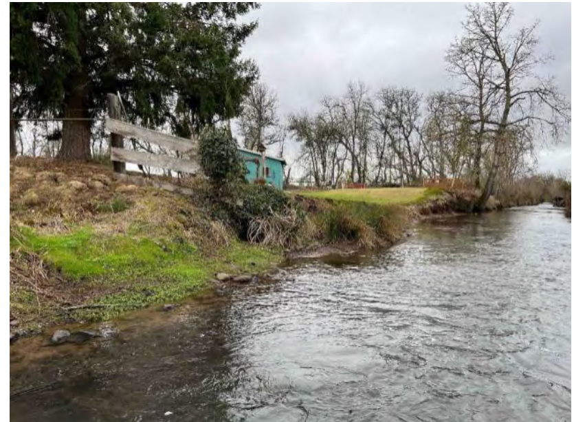
Photo 2967: Left bank downstream of failure
