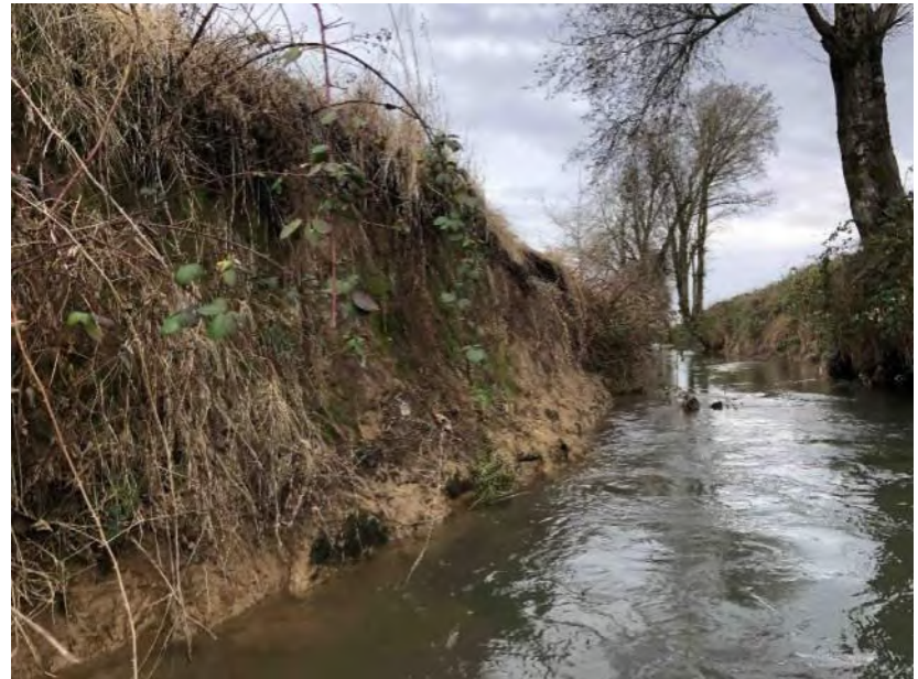
Photo 676: Upstream toward right bank
