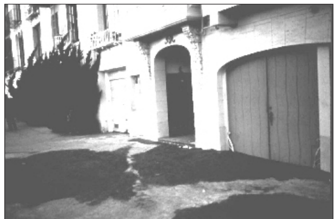
Figure 36 - Loma Prieta Earthquake, October 17, 1989. Lateral spreading, liquefaction and sand boils caused extensive damage in the Marina District of San Francisco, about 60 miles away from the epicenter.
