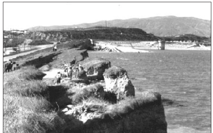
Figure 37 - Lower San Fernando Dam that was badly damaged by the 1971 San Fernando Earthquake.
