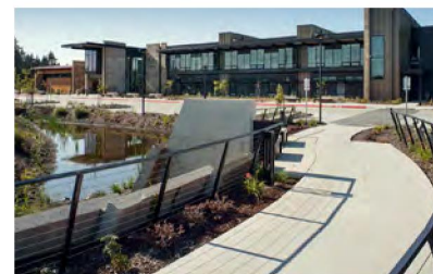
Light industrial and office facilities can take advantage of the natural creek corridors and water features in East Albany
