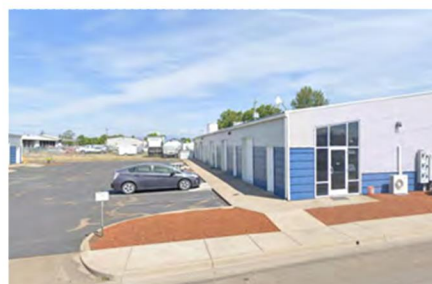
Light industrial and office building in East Albany study area
