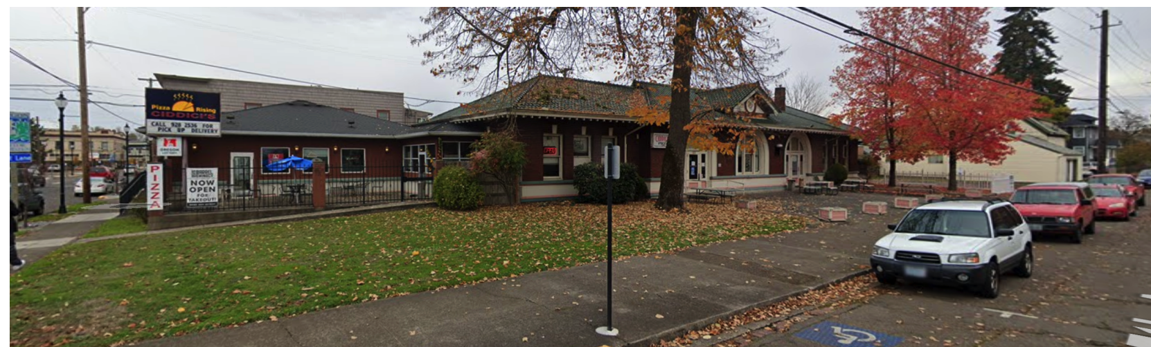
View of annex and connection to train station.
