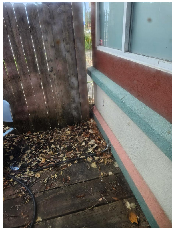
View of fencing at south annex connection which will be removed.
