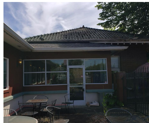
View of annex connection to be removed.
