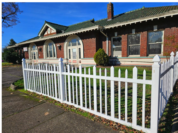
Exterior vinyl fencing to be removed.
