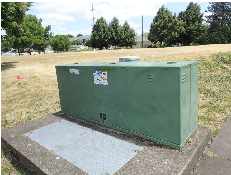
Pad-mounted transformer located in the southwest corner of the site.
